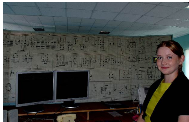
Figure 1: Control rooms changes from panels to screen
